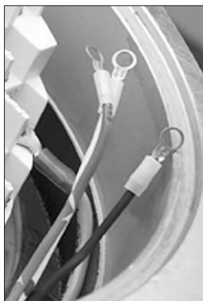
Figure 3.12 – Ring tongue connectors
